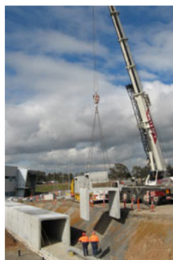
Last delivery of culverts under
