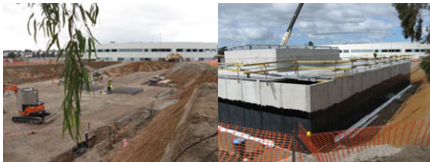
Then and now: excavation work in May, satellite building on September 4.
