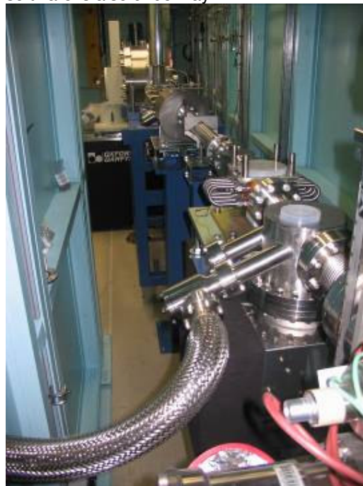
Looking downstream from right at the storage ring shield wall): the first ion pump, fixed mask, Bremsstrahlung collimator, white beam slits, white beam fluorescent screen and the double crystal monochromator installed and pumping down.
