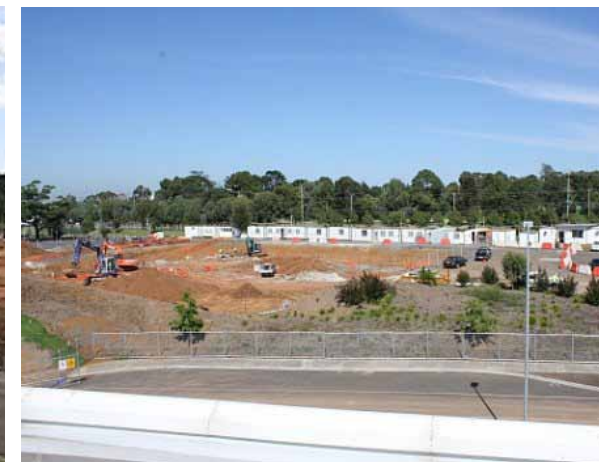
[15 February 2011]: construction work for NCCS building.
