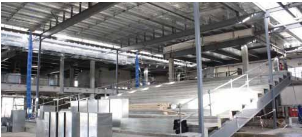
[12 August 2011]: the auditorium space inside the NCSS building.
