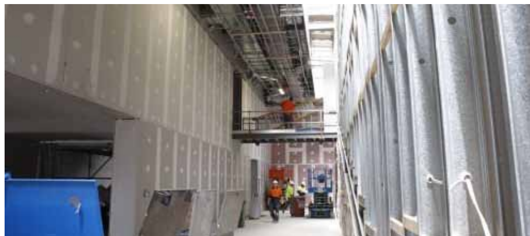
[14 October 2011]: inside the NCSS, looking south past the auditorium wall (LHS).
